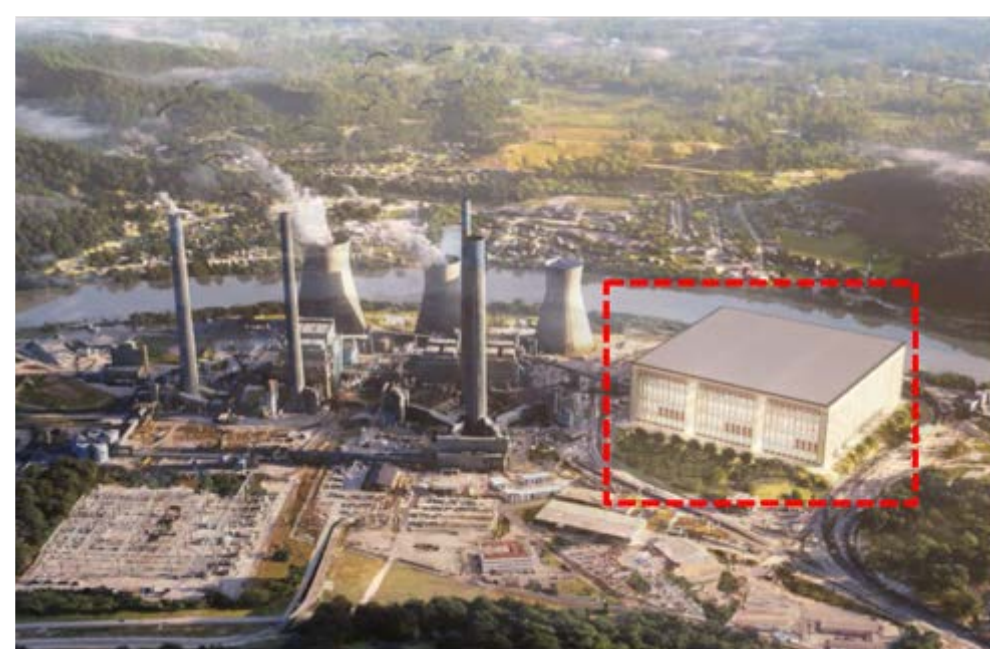
▲ Gravity Storage (Energy Vault)
