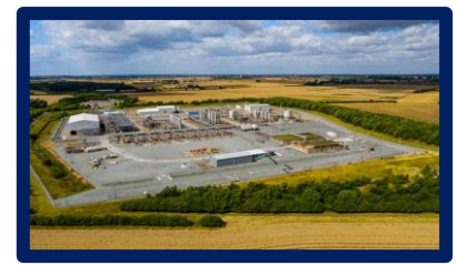
Aldbrough Hydrogen Storage
