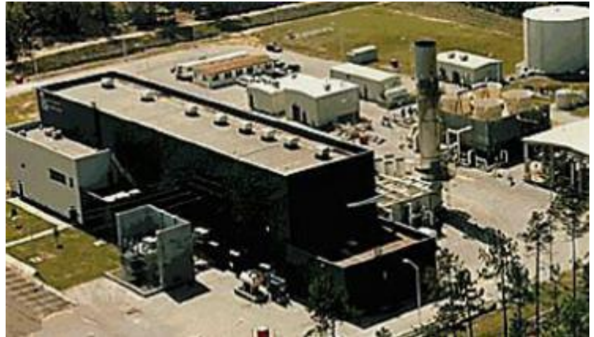
McIntosh USA (1991); 45-74 bar; 110 MW, 54% efficiency; Invest: $492/kW
