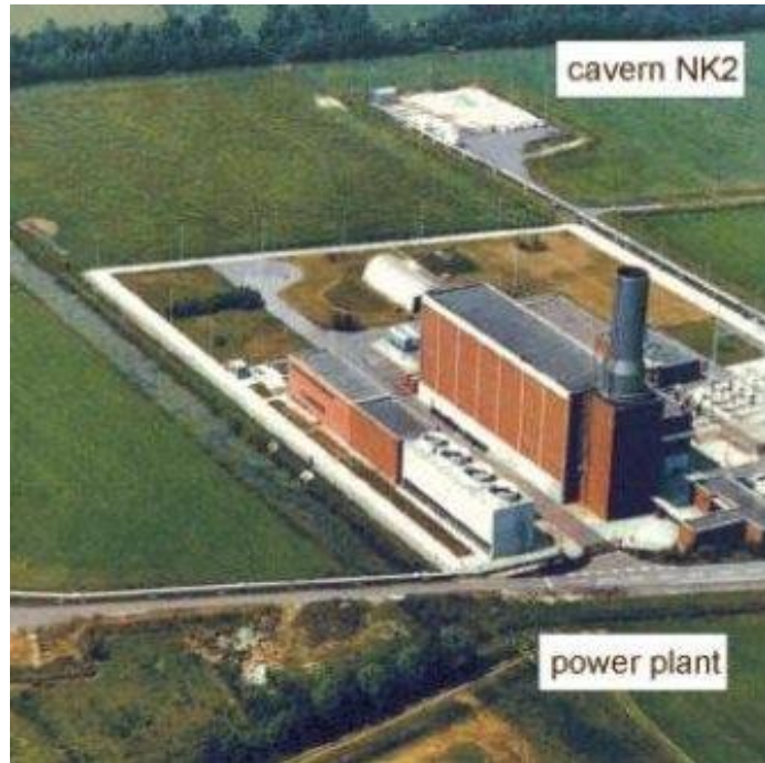
Huntorf Germany (1978). 20-43 bar; 290 MW, 42% efficiency; Invest: $480/kW
